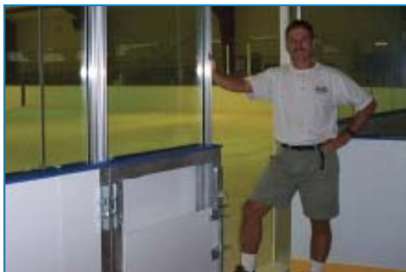
Rink Manager Mike Onorato explains how the backer panels, shown by him above, enhance the look of the facility. "The backer panels allow the mat flooring to be butted right up to the bottom of the board, and eliminates the collection of dirt and litter on the frame of the boards. They totally finish the look of the boards."
