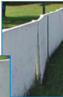
Typical damage to wood rink boards, which take time and materials to repair.
