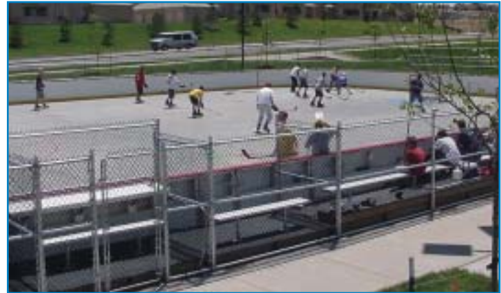
This rink in Cottonwood Park features a Border Patrol Pro 4000A dasher board system on an official-size concrete slab, and chain-link style penalty/player/scorer boxes with benches and elevated flooring
